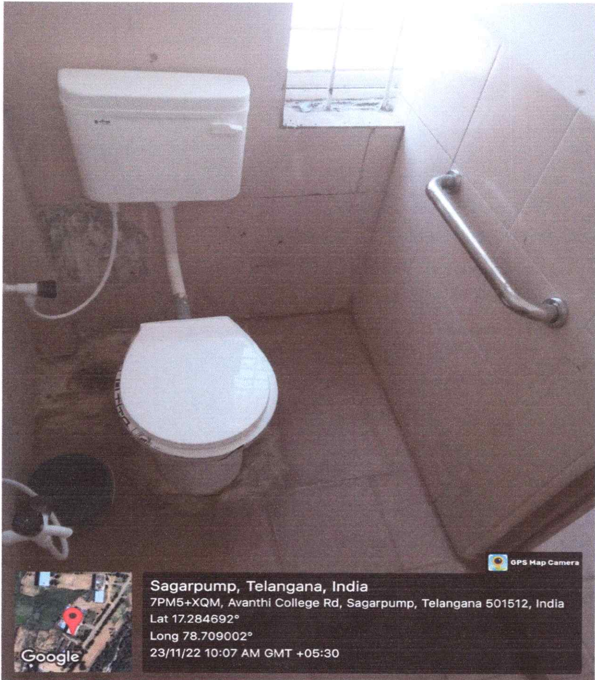
Divyangian-Friendly Washrooms In Main Block
