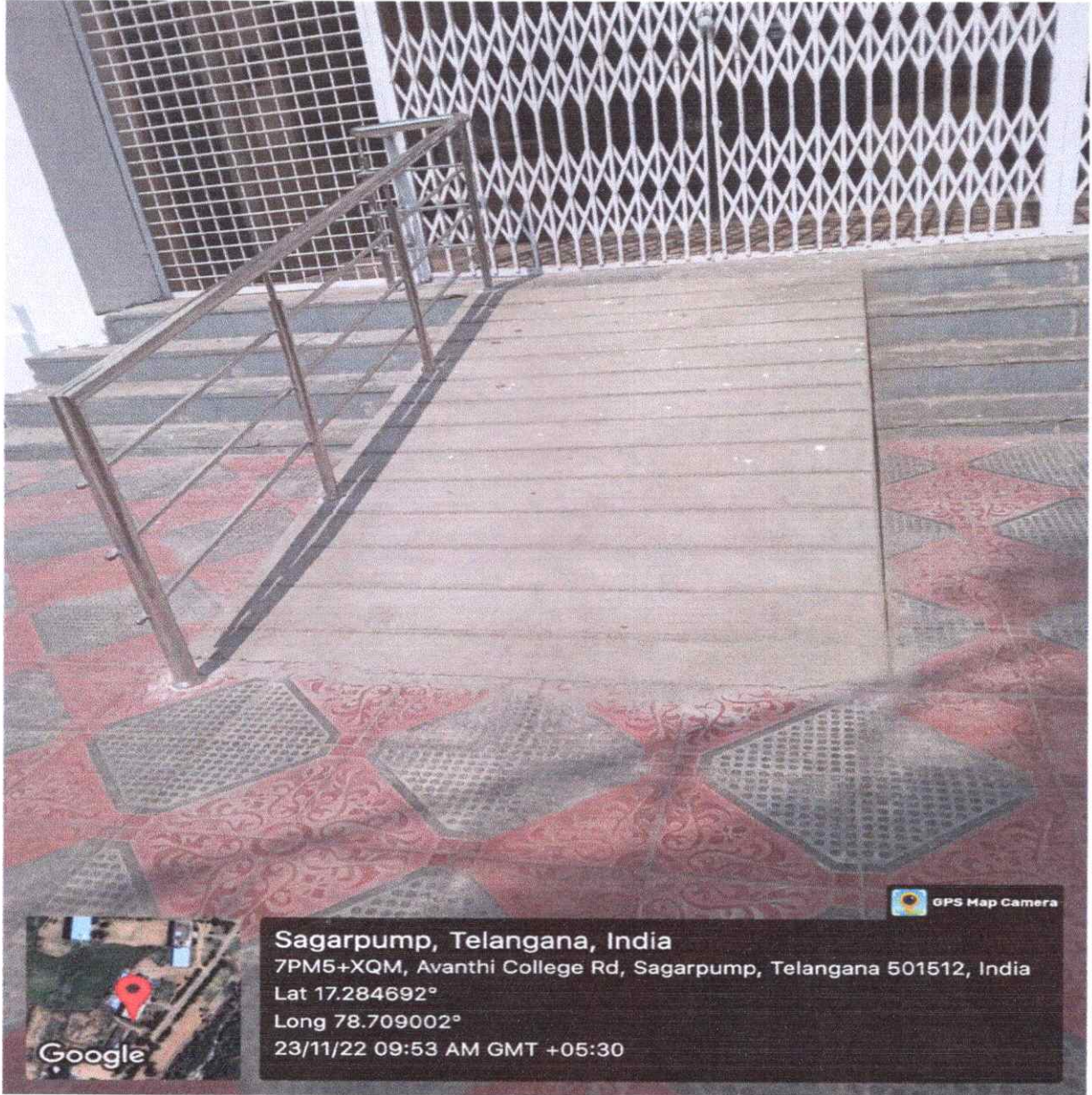
Ramps and railing for Physically Disabled at EEE Block
